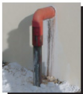
98% Sulfuric Acid Damages System in Florida Water Treatment Plant
